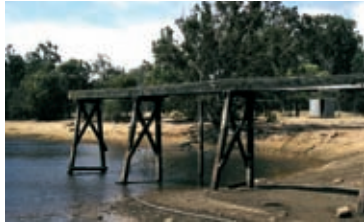
Kylie dam and water pipe support structure.
